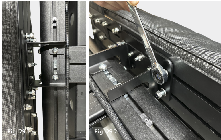
Tightening the nuts
