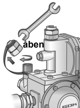
1. LUK GASUDTAGSVENTILEN PÅ GASBEHOLDERENS OVERLØBSSIKRING.
