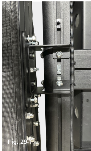
Tightening the nuts
